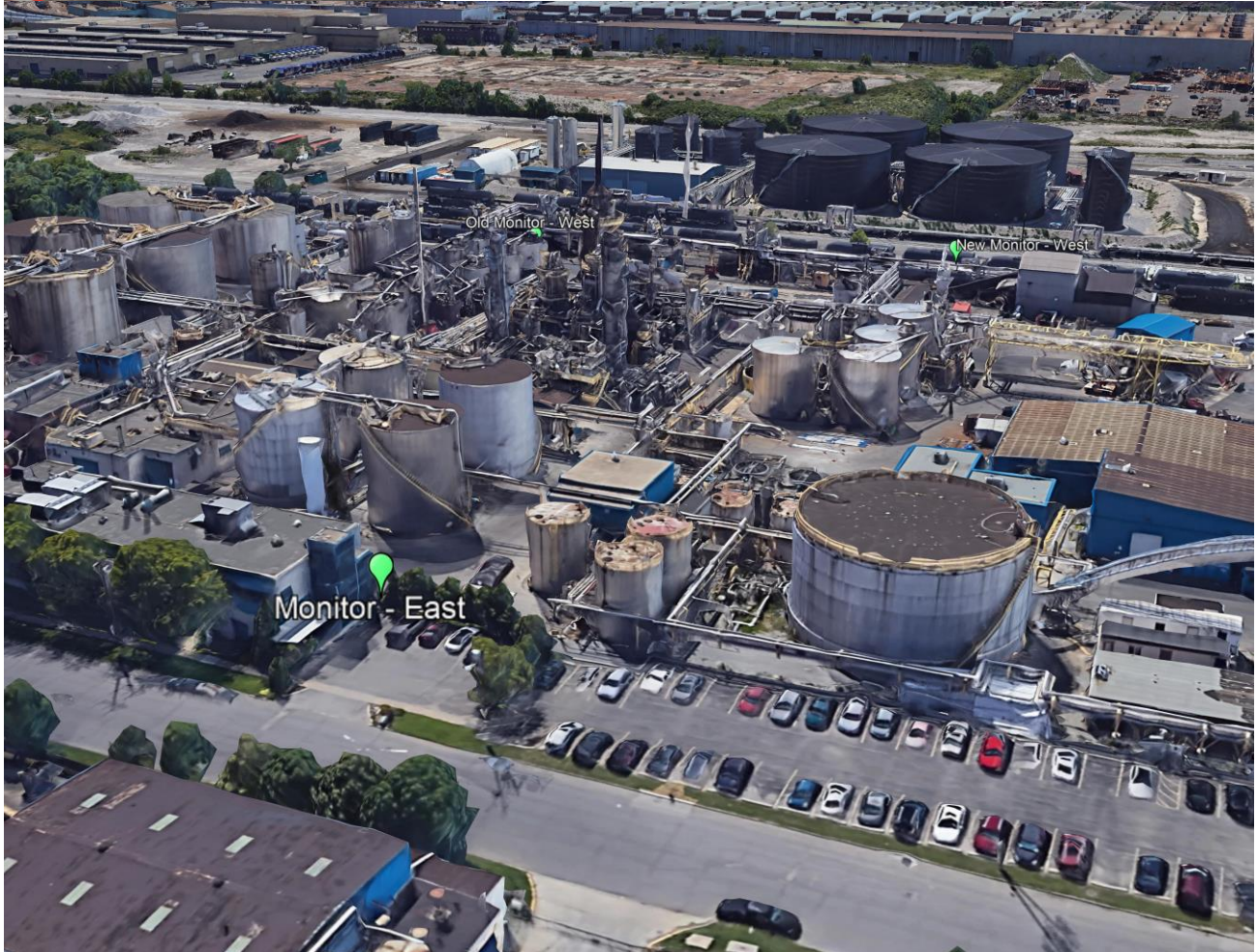
Figure A4: Aerial View 4 – East Monitoring Station
