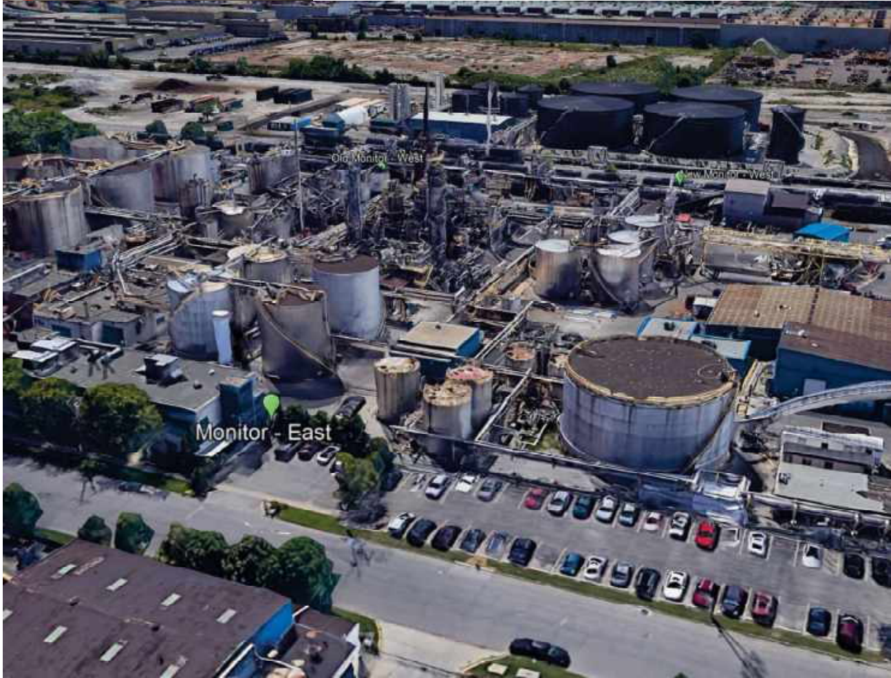
Figure A4: Aerial View 4 – East Monitoring Station
