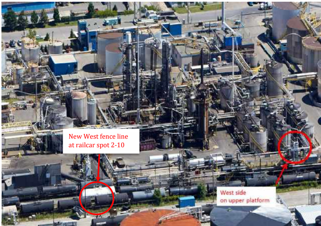
Figure 3: Monitor Locations on the West Side of the Facility
