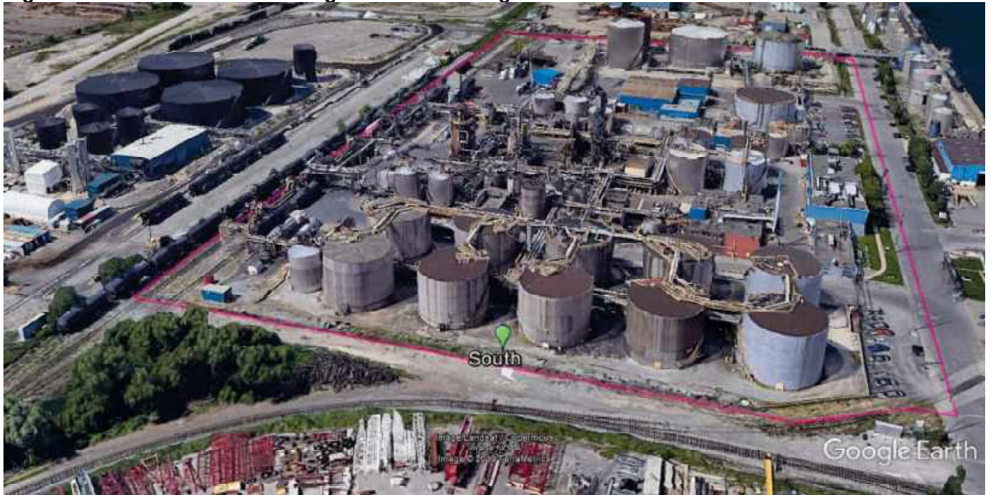
Figure A3: Aerial View 1 – Existing South Monitoring Station
