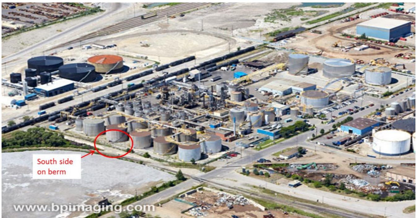
Figure 2: Monitor Location on the South Side of the Facility
