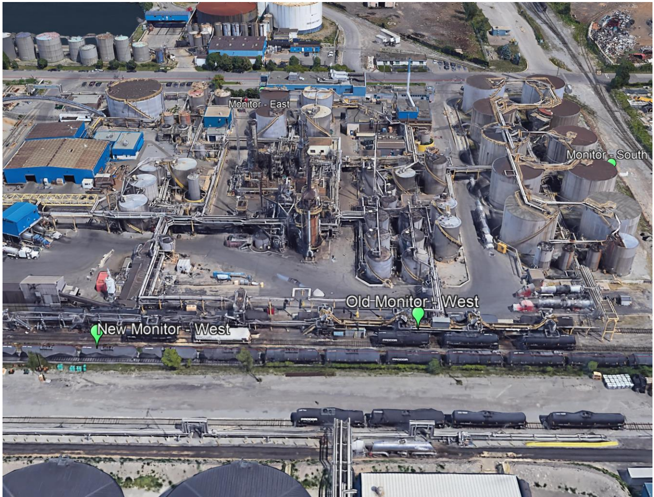
Figure A3: Aerial View 3 – New and Old West Monitoring Stations
